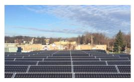
The solar system was designed using tenK Solar, a ARRA compliant solution with a low voltage design that optimizes the High School's rooftop space while delivering the highest reliability and safety standards. The tenK Solar system utilizes reflected light energy through reflectors that capture available light and reflect it back on the modules. In addition to increasing the yield of the system by up to 20%, the reflector has the added benefit of improving system aerodynamics.
